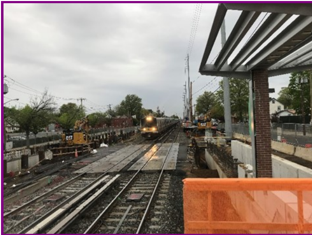
Rail road crossing and pedestrian underpass at South 12th Street
