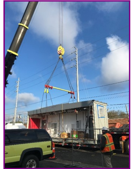
Installation of the materials delivered at the G-14 Electrical Substation
