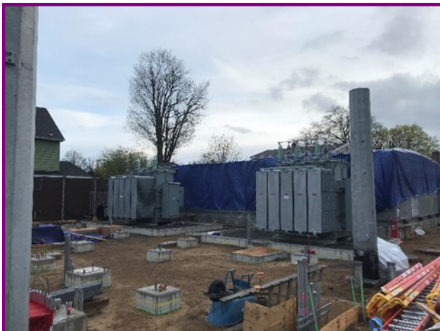
Construction site at the G-14 Electrical Substation
