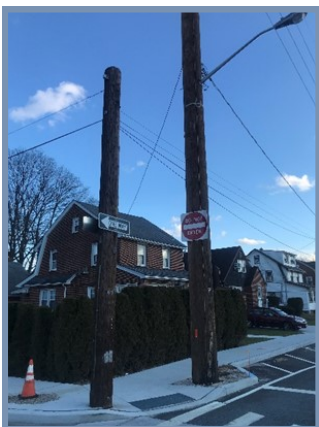
Relocation of cables from the Old Utility Poles to the New Utility Poles
