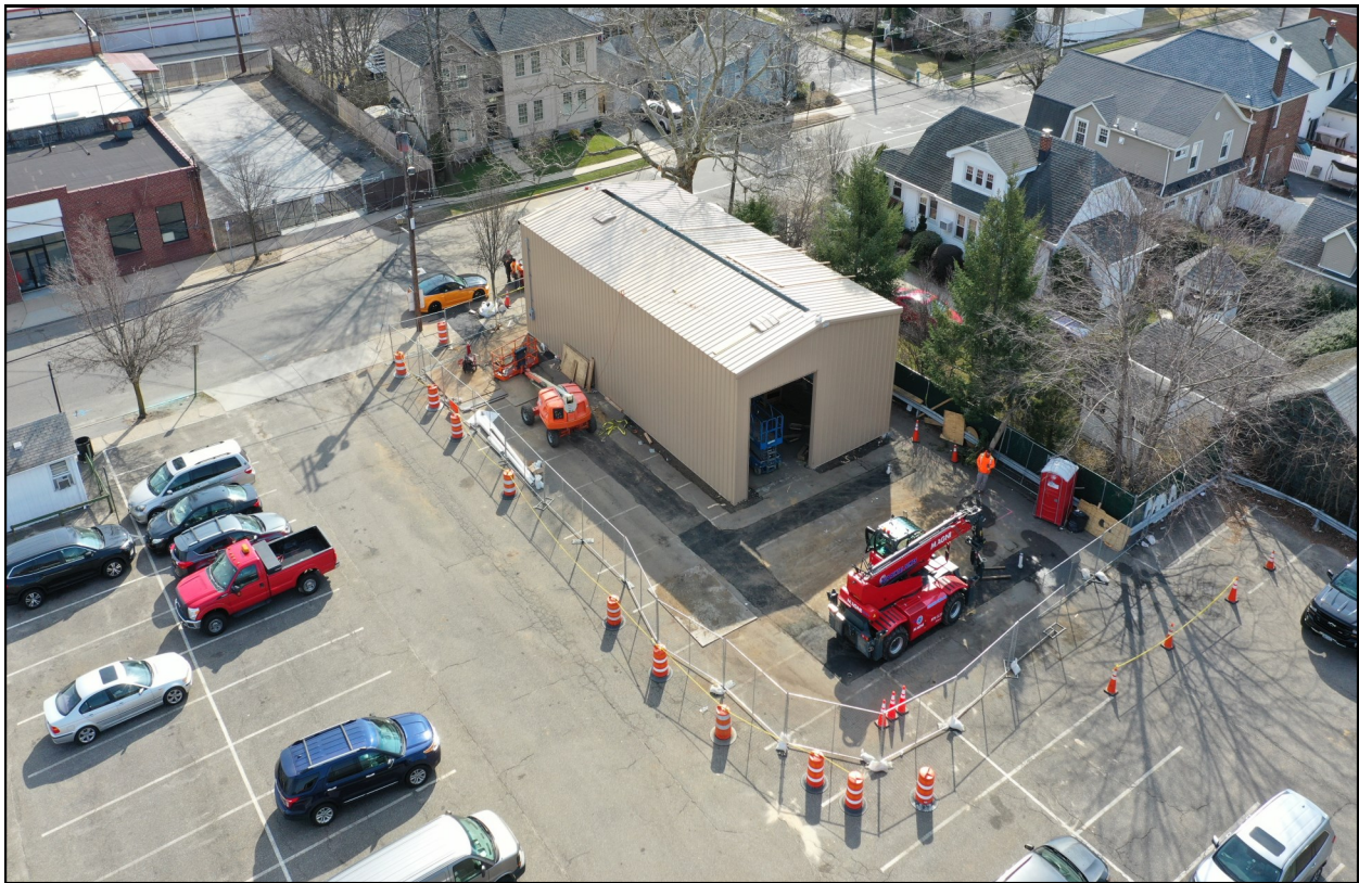
An aerial view of the new temporary fire facility that was set up in the South 12th Street Resident Parking Lot to provide emergency services to residents on the south side of the track during the LIRR Mainline Construction Project.
