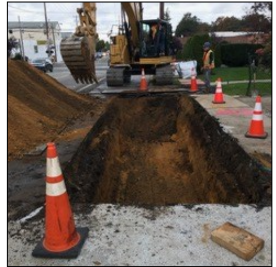
Excavation on Covert Avenue (looking north) for the installation of new sanitary drainage.
