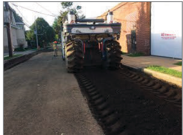
This machine pictured on South 2nd Street is mixing and injecting oil onto the roadway.
