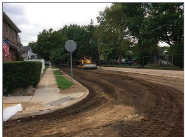
Final grading is done on Lincoln Avenue at Central Blvd. This is the final step before asphalt resurfacing.
