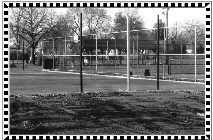
Final grading is the last step before asphalt paving.
