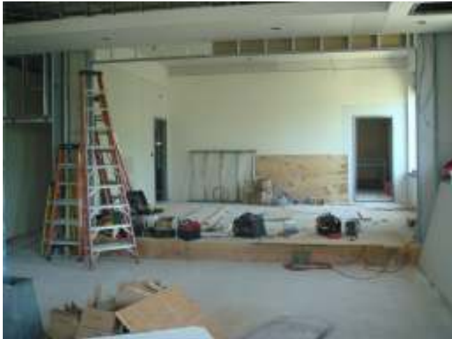
The new stage is taking shape.
